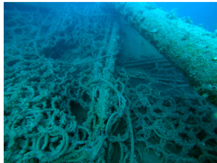
D: Netting attached to steel beams with spar B in the background
