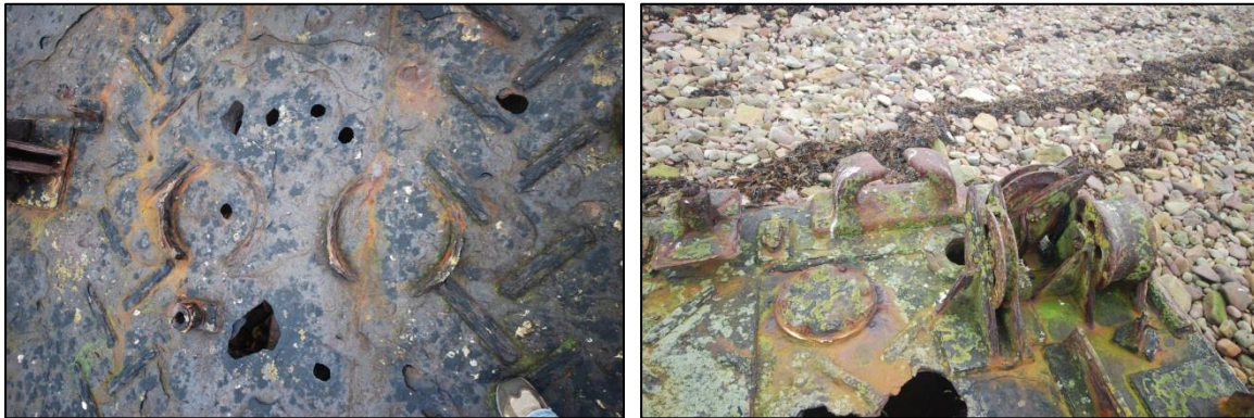
PLATE 17: EVIDENCE OF BURNING INDICATING SALVAGE OF MACHINERY
